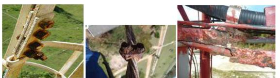
Figure (1): Effects of the coastal atmosphere on the corrosion of components in metal structures
