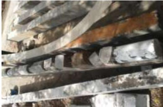
**Fig.5 Placing of Laminate over the Beam Soffit**
