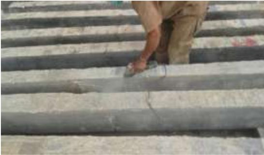
**Fig.3 Surface Preparation at Soffit of Beam**
