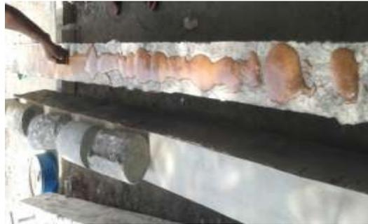
**Fig.4 Application of Epoxy Adhesive on Beam Soffits**
